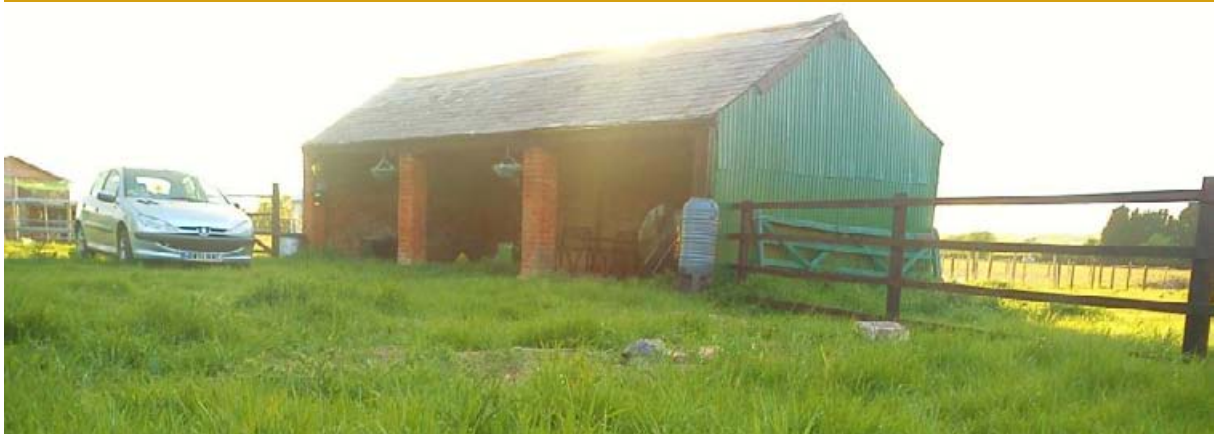
Open fronted brick barn with felt and slate roof measuring approx. 10.2 x 4.2 metres
