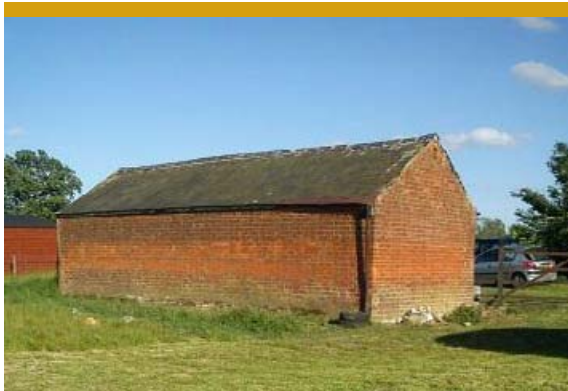
Rear of the brick barn
